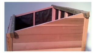
Step 14: Using 1 x 75mm tek screw , screw bottom purlin to top plate centrally in shed. Repeat with top purlin.
