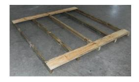
Step 2: Lay out remaining floor boards. Measure diagonals to ensure measurements are equal (I.e. floor is square). Rip down last floor board to suit gap, and nail off floor with 50mm flooring nails (10 nails per board).
