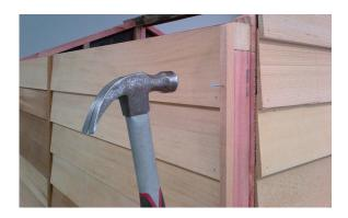
Step 12: Silicone and nail corner clashings on all corners as shown using 5 x beading nails per clashing.
