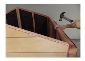
Step 9: Using 30mm clouts nail top cedar boards to stiffeners (2-3 per board). Predrill holes to stop boards from splitting.
