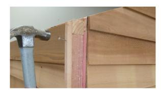
Step 12: Silicone and nail corner clashings on all corners as shown using 5 x beading nails per clashing.
