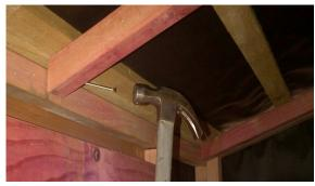
Step 18: Using 6 x 75mm tek screws, screw 3x collar ties to underside of rafters. Predrill before screwing if necessary.
