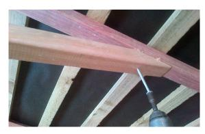
Step 19: Attach a plywood gusset to each side of rafters as shown using 8 x 30mm clouts per side.
