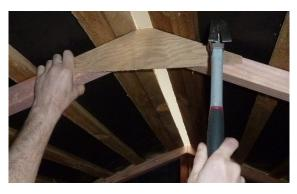
Step 20: Rivet ridge flashings together and attach to roof panels with 30mm clouts nailing into top purlin at approx 300mm centres.
