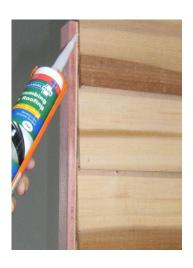
Step 7: Silicone and nail remaining beads on each panel. Screw panels together using 3 tek Screws per join and 4 on the longer joins on gable end panels.
