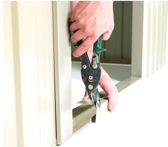
**Step2:** Measure and cut Doorstep Flashing (106) to fit in between Door Jambs. Position the Doorstep Flashing in between the Door Jambs at bottom of doorway, nail through top of flashing using five 30mm Clouts. Repeat with the Overdoor Flashing (105).
