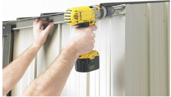
**Step 2:** Hang door in Door Track. At the right hand end of Door Track, adjust up or down so that the Door hangs parallel with shed. Fit one rivet at right hand end to hold in place. Repeat with left hand end of track.
