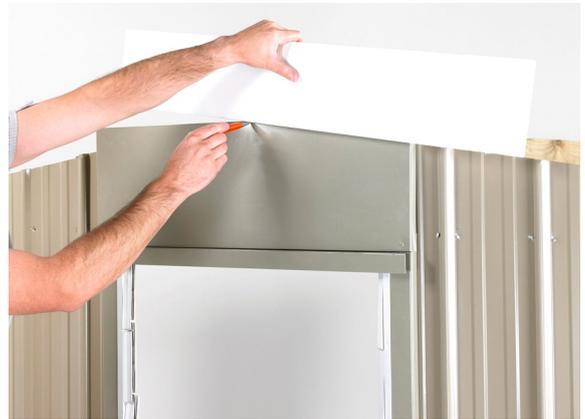
**Step 4:** If the Window is in the gable end, temporarily position the Over Panel above Window Frame. Following the same angle as the gable, mark and cut to suit.
