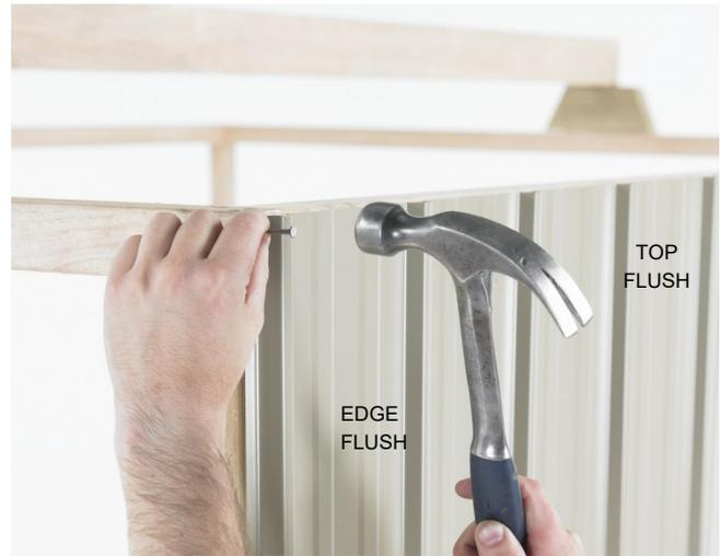
**Step 2: Back Wall:** Position the first Wall Sheet with the LIP on the right hand side. Ensuring the LIP is flush with the side of the Studs and the top of the Wall Sheet is flush with the top of the Top Plate, tack in place. Position the next Wall Sheet with the LIP on the right hand side. Overlap as shown in (fig 1). Ensuring Wall Sheet is flush with top of Top Plate, tack in place. Repeat with remaining sheet.
