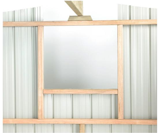
**Step 2:** On the inside of the shed, position studs and Nog centrally on window opening. Make sure the studs are parallel and nail into Top Plate and End Wall Nog.
