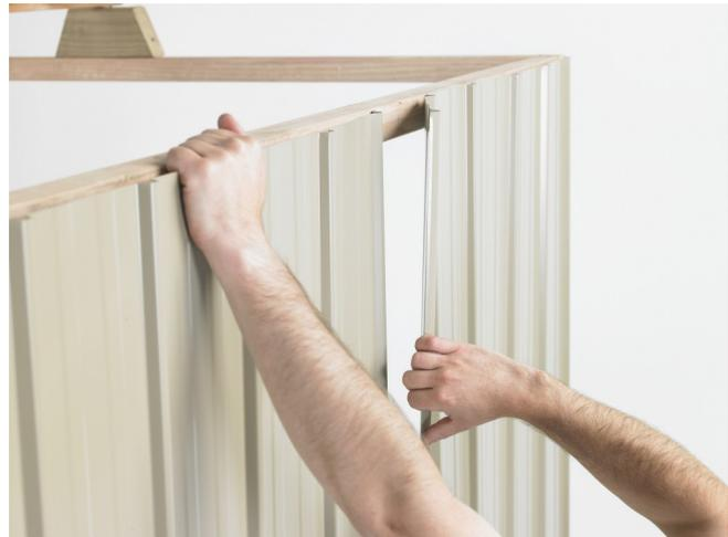
**Step 3: End Walls:** Lean Gable Wall Sheets against the shed to form gable shape. With the LIP flush with side of Stud tack in place ensuring the bottom of the Wall Sheet is 10mm above the bottom of the Bottom Plate. Tack on remaining Wall Sheets. Repeat with other gable end. If fitting a window, nail in Window Studs and Nog now. Refer to Window instructions.
