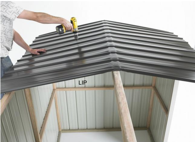
**Step 2:** Position first Roof Sheet centrally over Ridge Beam on the right hand end of shed with the LIP on the left hand side. (For sheds with a Clear Roof Panel, go to the next page). Position the next Roof Sheet. Ensure it overlaps correctly then rivet together, 100mm and 600mm down from the centre on both sides. Fit remaining Roof Sheet.
