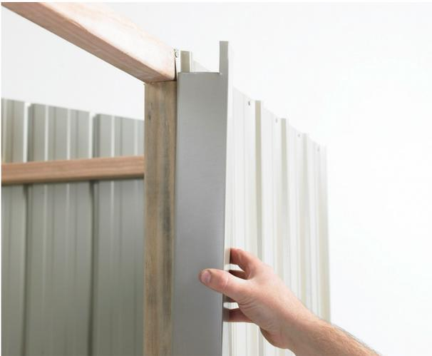
**Step1:** Fit Door Jamb Flashing (104) in between Top and Bottom Plates and hard against Stud. Attach Door Jamb Flashing with three rivets into Rib on the outside and three 30mm clouts into studs on the inside. Repeat with the other Door Jamb.
