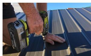
Note. Use 50mm Roofing screws with washers for bottom purlin and 30mm clouts for top purlin.
