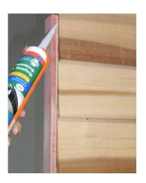
Step 7: Silicone and nail remaining beads on each panel. Screw panels together using 3 tek Screws per join and 4 on the longer joins on gable end panels.
