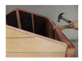
Step 10: Using 30mm clouts nail top cedar boards to stiffeners (2-3 per board). Predrill holes to stop boards from splitting.
