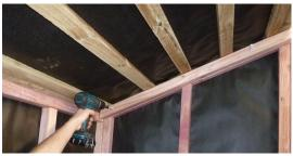
Step 15: Using 2 x 75mm framing nails, nail centre rafter to front and back top plate stiffeners. Predrill if necessary.
