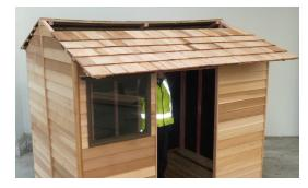
Step 14: Using 75mm tek screws, screw roof panels into end wall panels, (2 screws each end per panel), ensuring end of rafter lines up with centre of gable panel.
