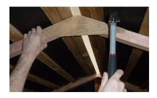
Step 17: Attach ridge flashing to shingle roof panels with 30mm clouts nailing into top purlin at approx 500mm centres.
