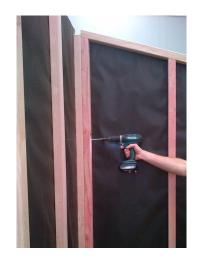
Step 6: Silicone edge of weatherboards on standing panel and nail on cedar beads with 5 x bead nails. (Refer to wall plan for correct beads).
