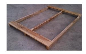
Step 2: Lay out remaining floor boards. Measure diagonals to ensure measurements are equal (i.e. floor is square). Rip down last floor board to suit gap, and nail off floor with 50mm flooring nails (10 nails per board).
