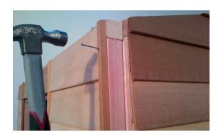
Step 12: Silicone and nail corner clashings on all corners as shown using 5 x bead nails per clashing. Note short clashings at the front, long clashings at the rear.
