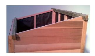
Step 14: Using 1 x 75mm tek screw, screw bottom purlin to top plate centrally in shed.
