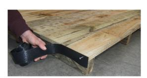
Step 4: Unpack panels and identify wall panels and door positions as per plan on following page.Select two panels that go either side of a corner (i.e. end and standard panel) and stand together.
