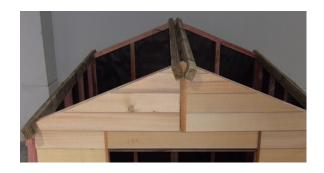
Step 14: Using a 75mm tek screw, screw bottom purlin to top plate centrally in shed.
