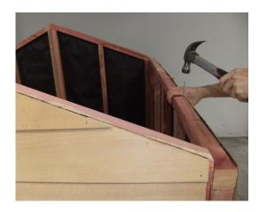
Step 9: Using 30mm clouts nail top cedar boards to stiffeners (2-3 per board). Predrill holes to stop boards from splitting.
