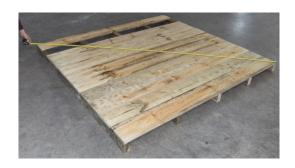
Step 3: Nail plastic weatherstrip to edge of floor on all four sides, with 30mm clouts, (approx 5 nails per side) ensuring top edge is flush with top of floor. This isn't required if shed is on a concrete base.
