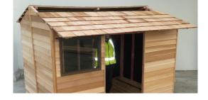
Step 14: Using 75mm tek screws, screw roof panels into end wall panels, (2 screws each end per panel), ensuring end of rafter lines up with centre of gable panel.
