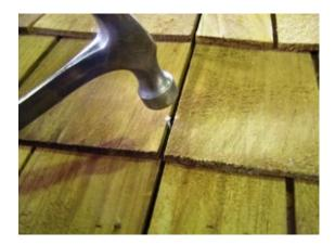
Step 22: Nail using 50mm nails, above the bottom of the next row of shingles.
