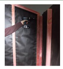
Step 6: Silicone edge of weatherboards on standing panel and nail on cedar beads with 5 x bead nails. (Refer to wall plan for correct beads).
