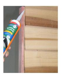
Step 7: Silicone and nail remaining beads on each panel. Screw panels together using 3 tek Screws per join and 4 on the longer joins on gable end panels.
